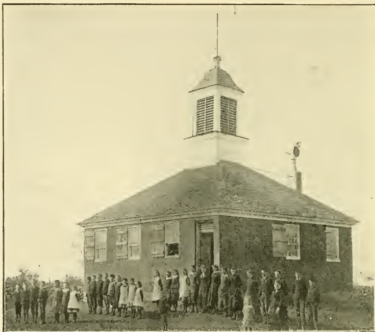
THE FIRST SCHOOLHOUSE AT RYE CENTER.
